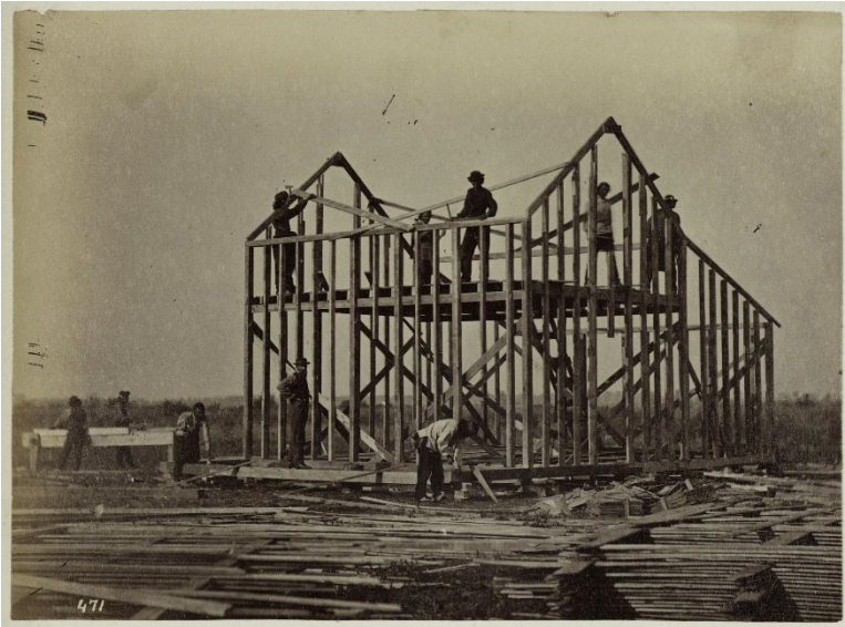
Figure E: William Henry Jackson, “[Omaha] Indian Carpenters Building Houses for the Tribe,” Photograph c1868. Princeton University Library, Special Collections: Photographs of North American Indians, 1840-1879 , https://findingaids.princeton.edu/catalog/WC054_c00491 (accessed June 2021).
